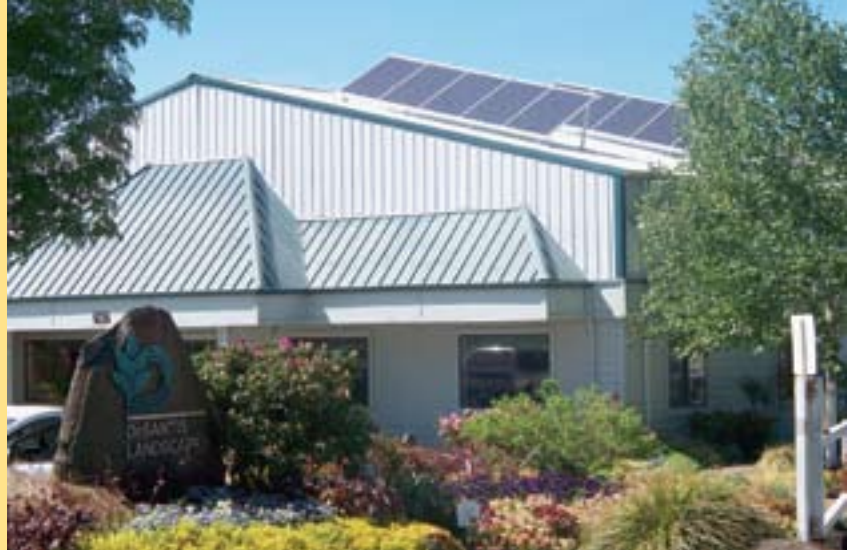
The DeSantis Landscapes Corporate Headquarters’ 3.8KW solar photovoltaic array provides over 15 percent of the office’s energy needs.
